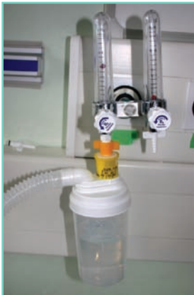
Humidification system for oxygen
